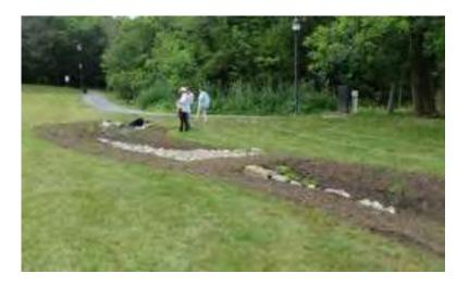
Vegetated Stormwater Conveyances serve to prevent scour and erosion and provide water quality treatment while conveying stormwater. They are constructed trapezoidal or parabolic channels lined with vegetation that inhibits erosion. From a water quality perspective, they are preferable to pipes because they allow more soil/water contact and more opportunity for infiltration. There are three types of vegetated conveyances: Dry Swales, Step Pool Conveyance, and Wet Swales.
