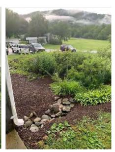
A Rain Garden is a shallow landscaped depression that temporarily ponds stormwater runoff and encourages it to infiltrate into the underlying soil. Rain Gardens are vegetative infiltration practices providing runoff reduction and pollutant removal.
