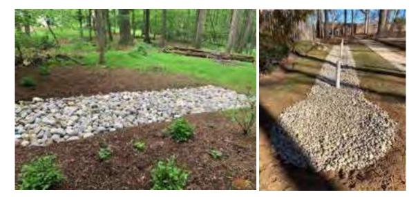
Infiltration practices provide temporary surface and/or subsurface storage of stormwater runoff until it seeps into the ground. Infiltration is a non-vegetative practice that provides runoff reduction. Surface infiltration trenches or basins may utilize a berm to pond runoff; subsurface trenches or basins store runoff in a gravel reservoir, open-bottomed chamber, or perforated chamber. Infiltration does not convey runoff like a French Drain.
