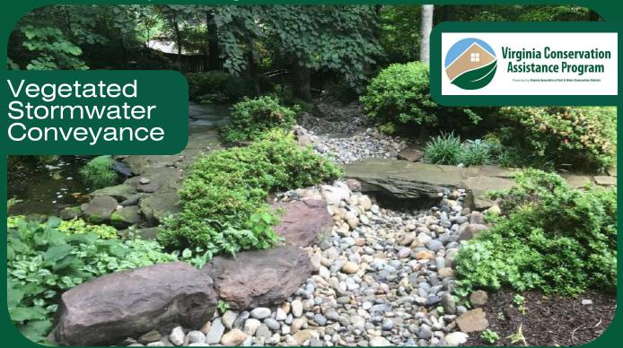
Vegetated Stormwater Conveyances serve to prevent scour and erosion in an existing channelized area and provide water quality treatment while conveying stormwater. They are constructed channels lined with vegetation that inhibits erosion. From a water quality perspective, they are preferable to pipes because they allow more soil/water contact and more opportunity for infiltration.
