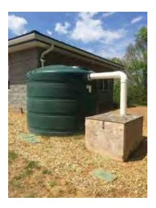
Rainwater Harvesting systems intercept, store, and release rainfall for future use. For purposes of this specification, Rainwater Harvesting includes the collection and conveyance of roof runoff into an above- or below-ground storage tank where it can be reused or safely diverted to a receiving area for infiltration.
