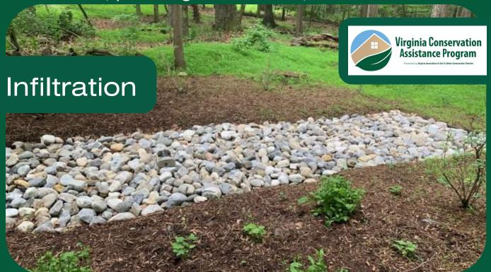
Infiltration practices provide temporary surface and/or subsurface storage of stormwater runoff until it seeps into the ground. Infiltration is a non-vegetative practice that provides runoff reduction. Surface infiltration trenches or basins may utilize a berm to pond runoff; subsurface trenches or basins store runoff in a gravel reservoir, open-bottomed chamber, or perforated chamber. Infiltration does not convey runoff like a French Drain.
