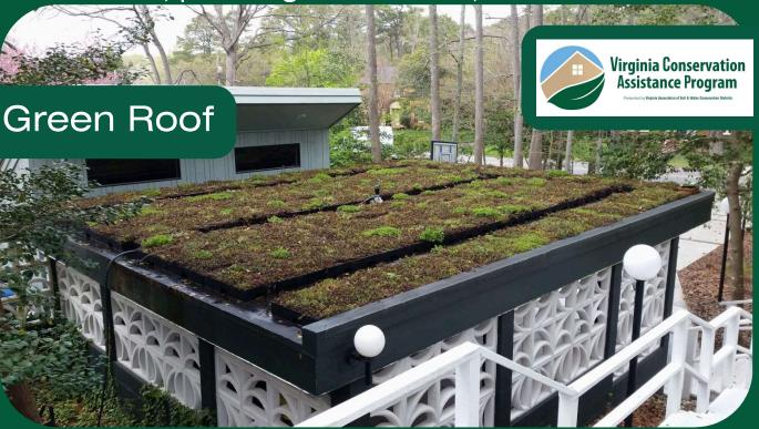
Green Roofs or vegetated roofs are alternative roof surfaces that typically consist of waterproofing and drainage materials and an engineered growth media that is designed to support plant growth. Vegetated roofs capture and temporarily store stormwater runoff in the growth media. A portion of the captured stormwater evaporates or is taken up by plants, which helps reduce runoff volumes, peak runoff rates, and pollutant loads on development sites.
