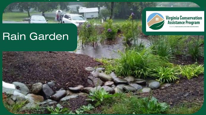
A Rain Garden is a shallow landscaped depression that temporarily ponds stormwater runoff and encourages it to infiltrate into the underlying soil. Rain Gardens are vegetative infiltration practices providing runoff reduction and pollutant removal.
