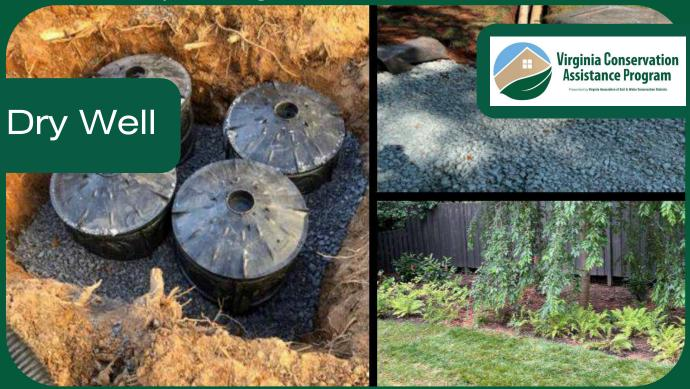
A dry well is a subsurface storage facility that temporarily stores stormwater runoff until it can seep into the surrounding soil. Runoff is stored in a reservoir of gravel, an open-bottomed chamber, or both.
