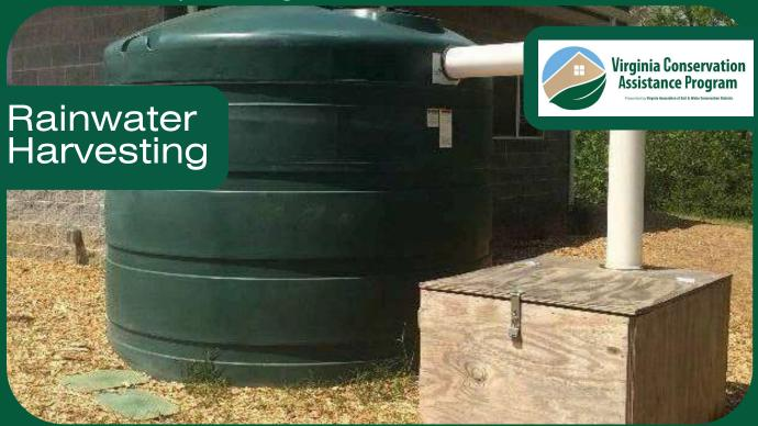
Rainwater Harvesting systems intercept, store, and release rainfall for future use. For purposes of this specification, Rainwater Harvesting includes the collection and conveyance of roof runoff into an above-or below-ground storage tank where it can be reused or safely diverted to a receiving area for infiltration.
