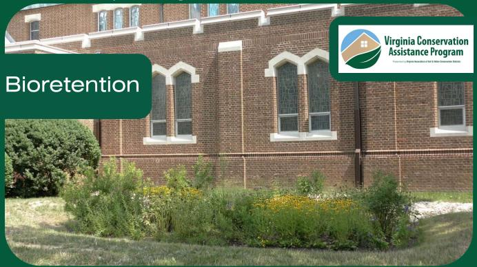
Bioretention is a shallow landscaped depression that temporarily allows runoff to pond and then filter through an engineered soil media prior to being discharged to an underdrain or absorbing into the underlying soil. Bioretention provides both runoff reduction and pollutant removal.
